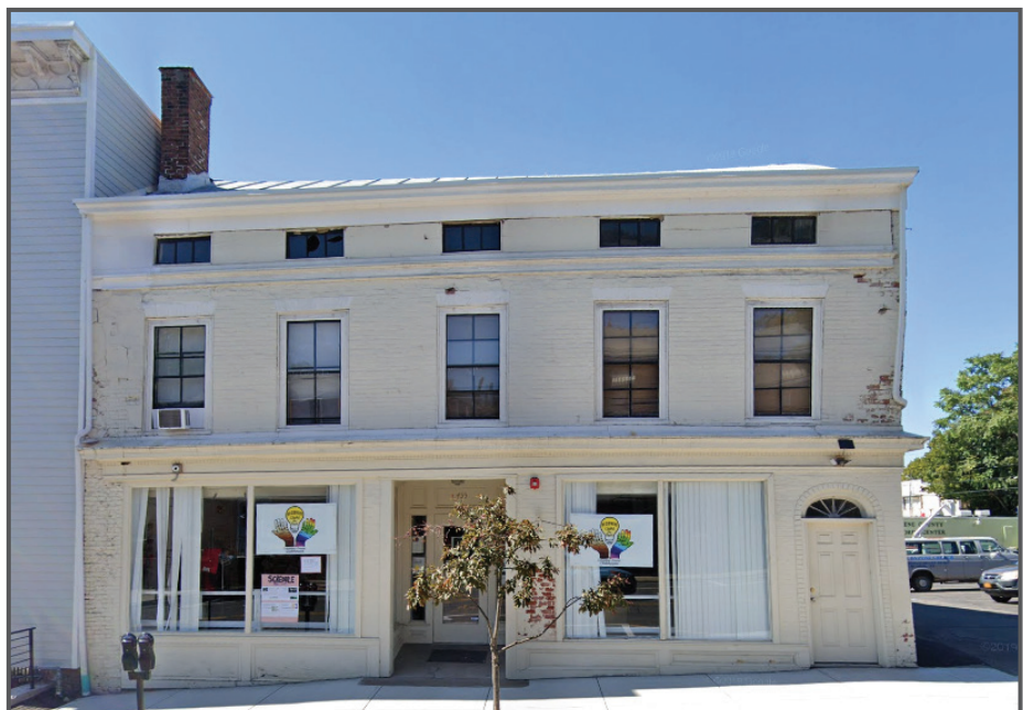
455 Main Street houses the Mental Health Association of Greene County, including its youth clubhouse along with crisis services and supportive housing. The structure requires several improvements to continue serving these populations.
